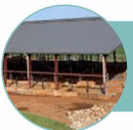
Livestock & Poultry Research Facilities (Various Locations)
