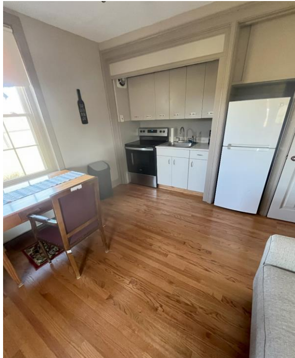
Annex Freeze Damage Repairs
